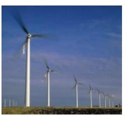
tricity. The 3-blade, variable pitch propeller used on the Z-750 (as this latest-generation turbine is called) measures 156 ft. in diameter, and weighs 34,000 lbs! The turbines are spread over 10 square miles of farmland.
