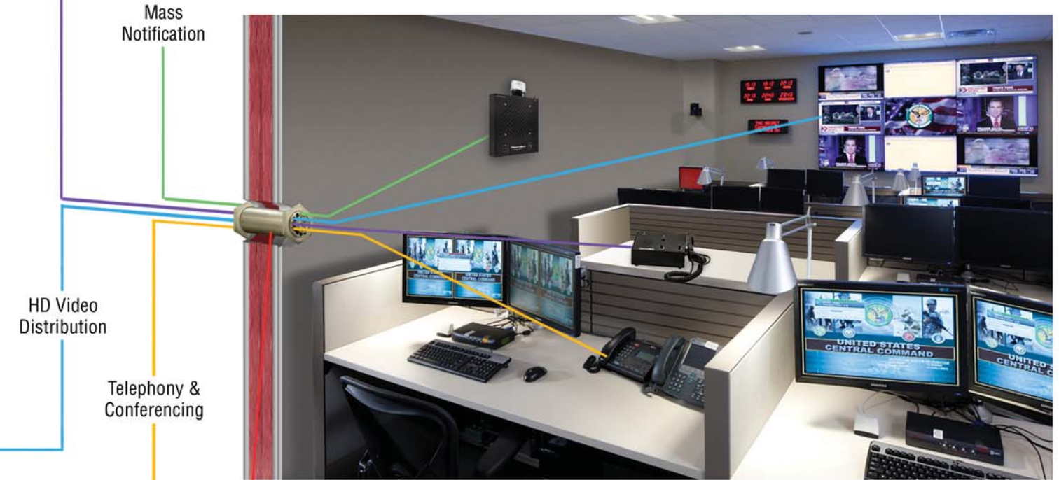
SCIF (Sensitive Compartmented Information Facility)
